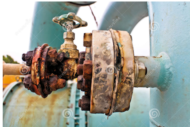
FIGURE 86: Check for corrosion in valves 104
