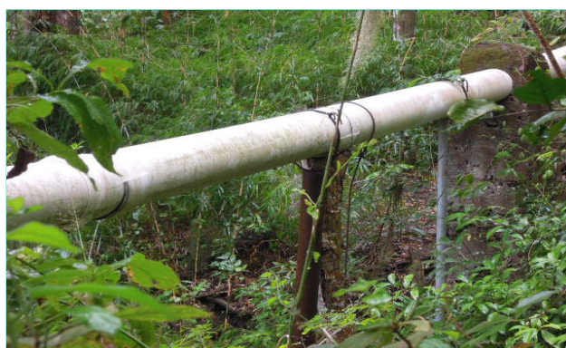
FIGURE 4: A PVC pipe penstock 4
