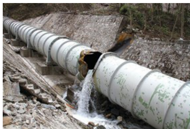
FIGURE 80: Damaged and leaking penstock 98
