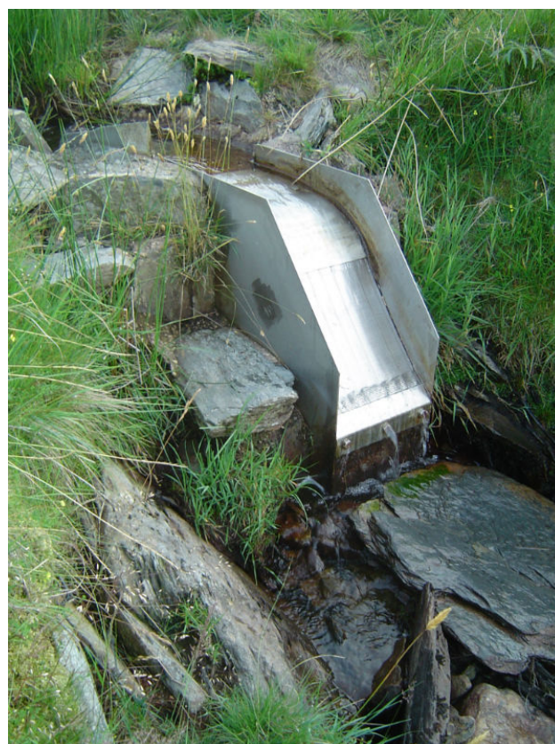
FIGURE 59: Filter installed with penstock outlet at bottom 78
