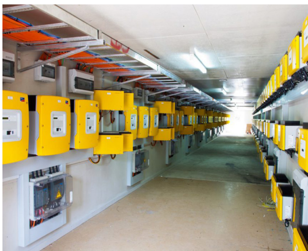
FIGURE 19: Sunny Island Inverters delivered by SMA control the standalone systems 42
