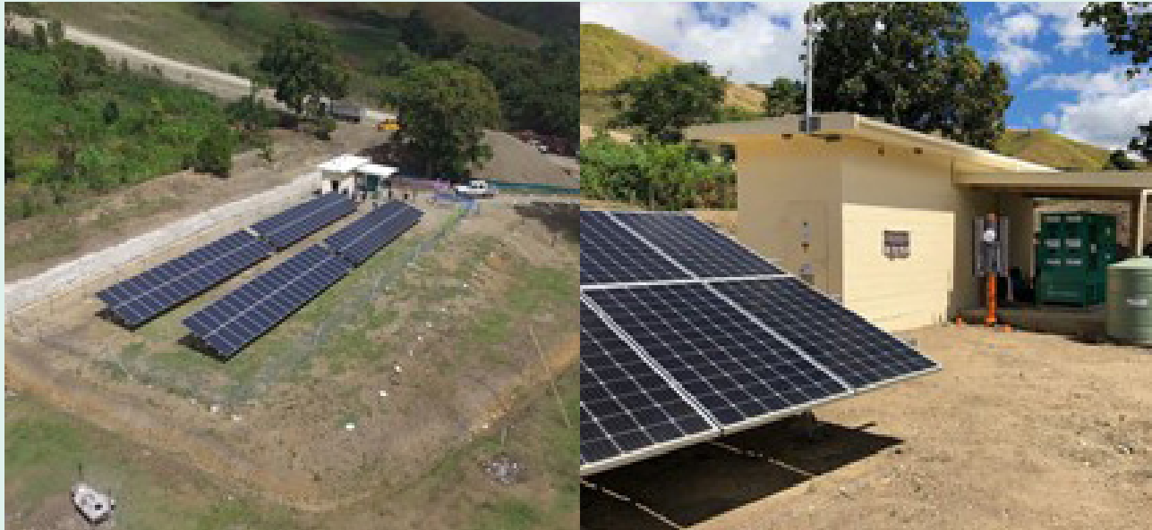
FIGURE 39: Nakoro Solar Mini-grid system
