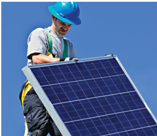
FIGURE 45: Wear a harness connected to a secure structure 48
