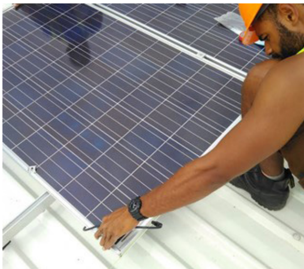
FIGURE 53: Solar panels mounted on rails 50
