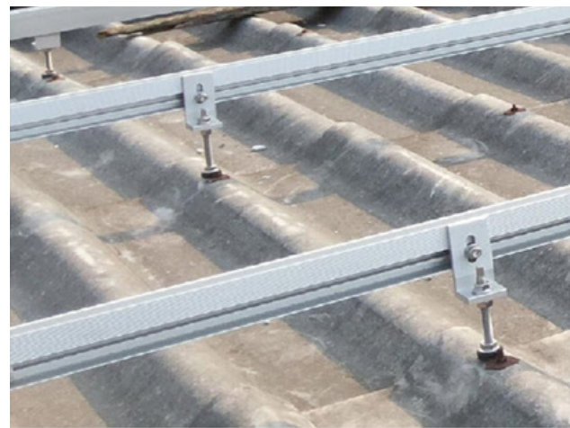
FIGURE 51: Solar Rails on corrugation 48
