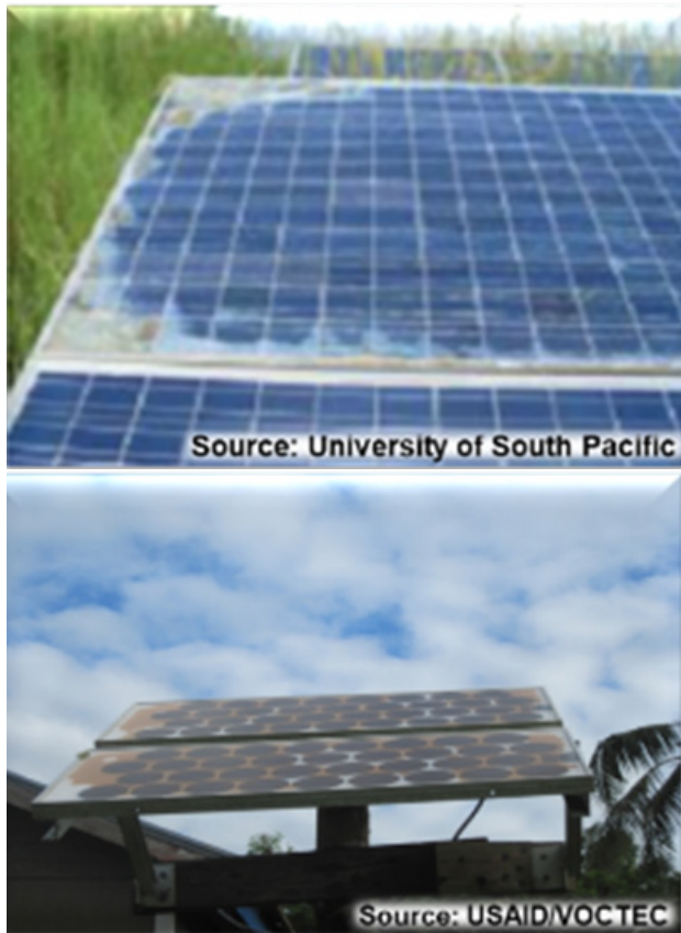
FIGURE 76: Panel Surface damage
