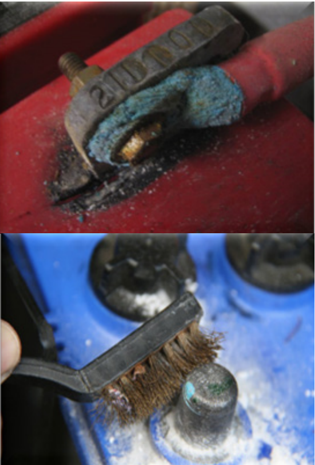
FIGURE 46: Cleaning Terminal Corrosion 54
