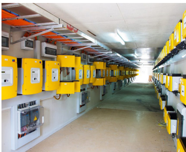
FIGURE 19: Sunny Island Inverters delivered by SMA control the standalone systems 41
