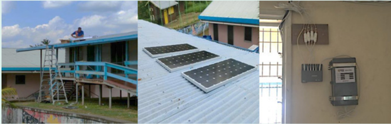
FIGURE 39: Installation of Solar Home System at Kwikila Health Centre in Central Province (left) – Technician mounting a Solar PV on the Rooftop, (middle) – Completed Simple Installation on the roof top, (right) – Simple Plug and play wiring showing Control Box and Battery Storage box 40
