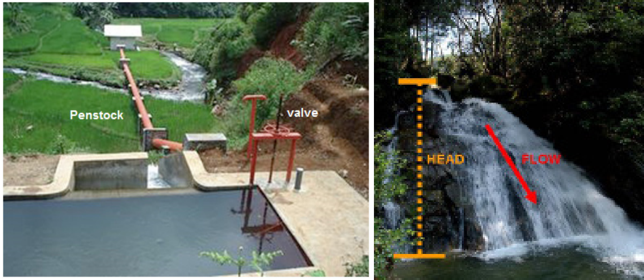
FIGURE 6: Schematic and pictures of a typical Pico-Hydro system 6
