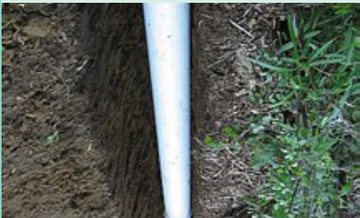
FIGURE 21: Penstock (PVC pipe) 21
