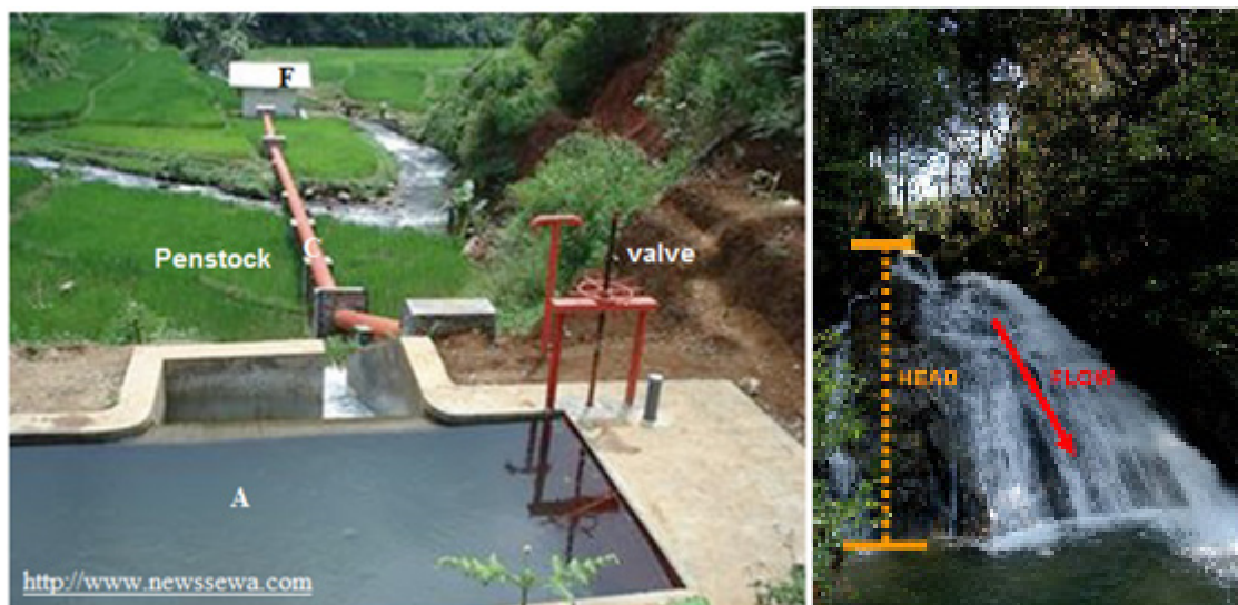
FIGURE 6: Schematic and pictures of a typical Pico-hydro System 6
