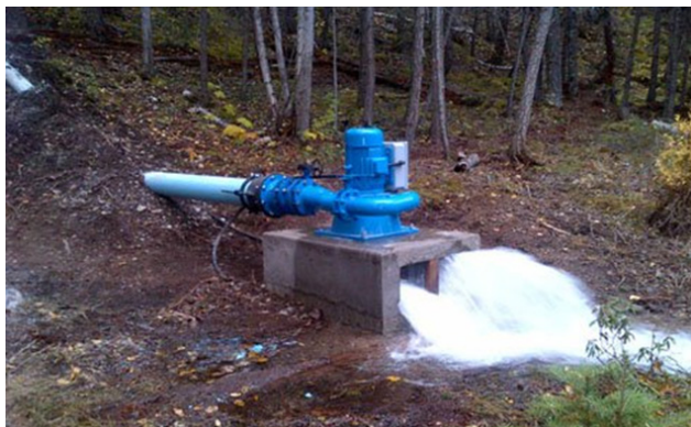
FIGURE 20: Micro -Hydro System 29
