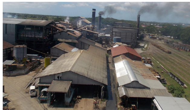
FIGURE 36: Sugar mill in Fiji - Burning sugarcane bagasse to generate electricity 43
