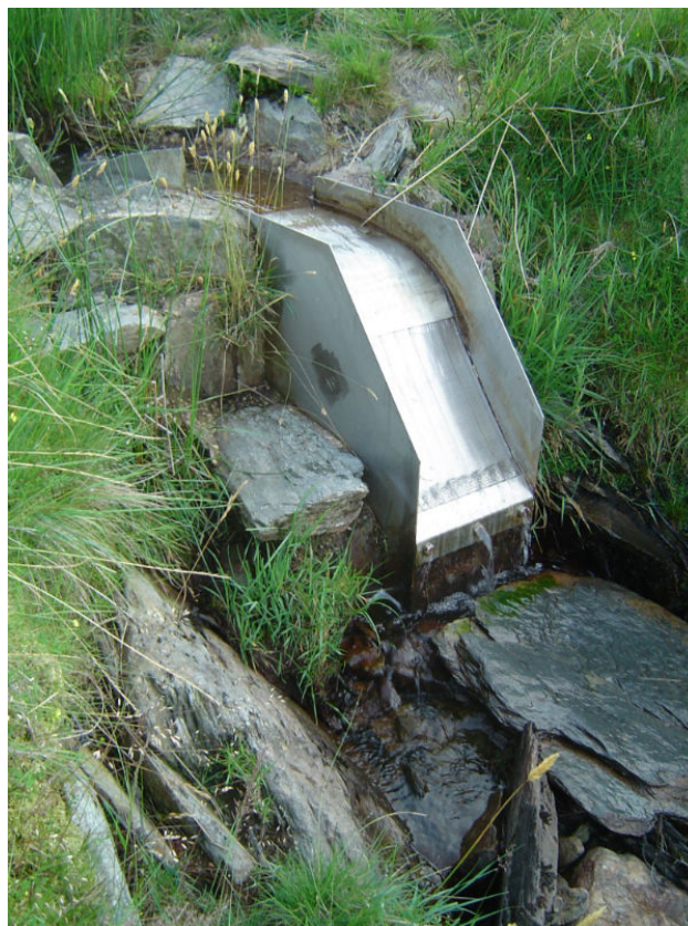
FIGURE 59: Filter installed with penstock outlet at bottom 78
