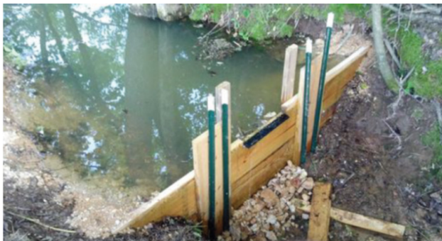
FIGURE 85: Stop-Log rack arrangement as a weir or dam to support forebay 103
