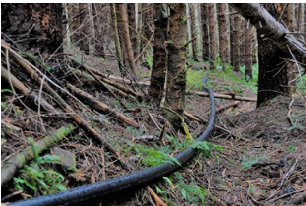
FIGURE 61: Penstock pipe 80
