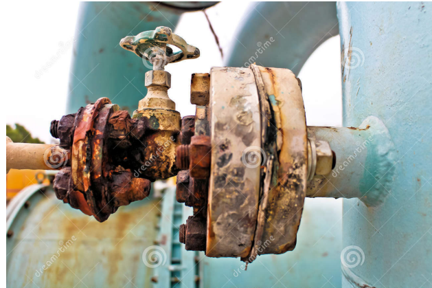
FIGURE 86: Check for corrosion in valves 104
